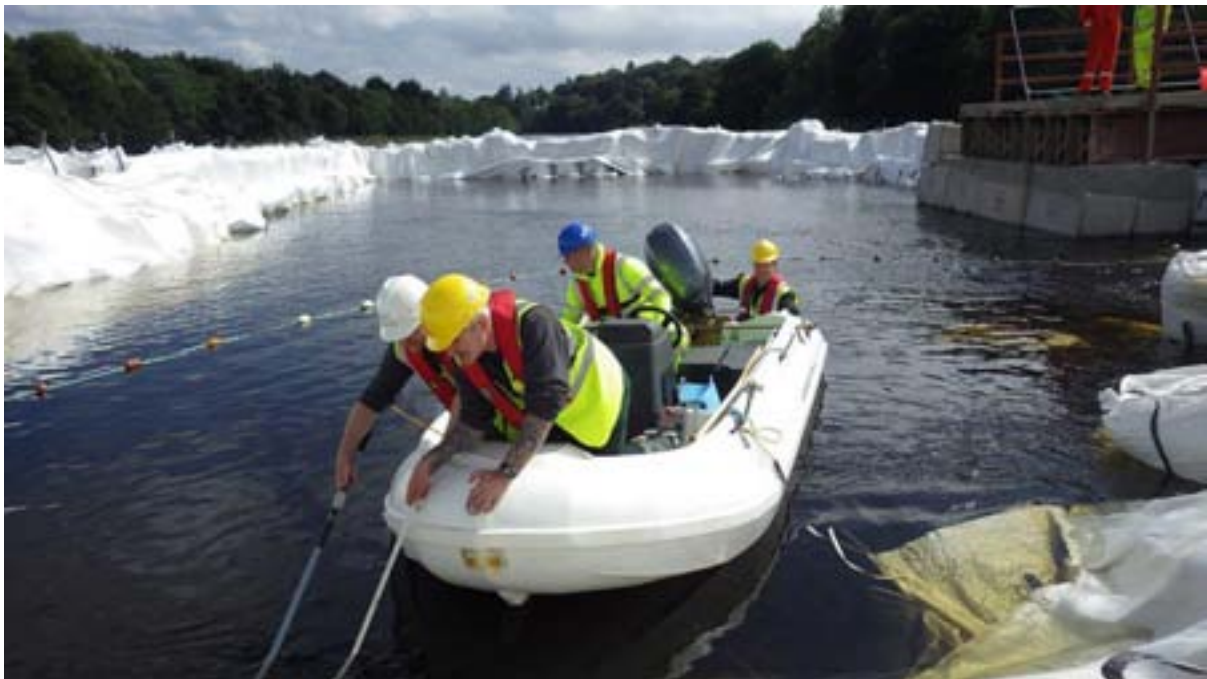
A fish rescue being completed by board and trust staff in the south pier of the West Link Bridge
